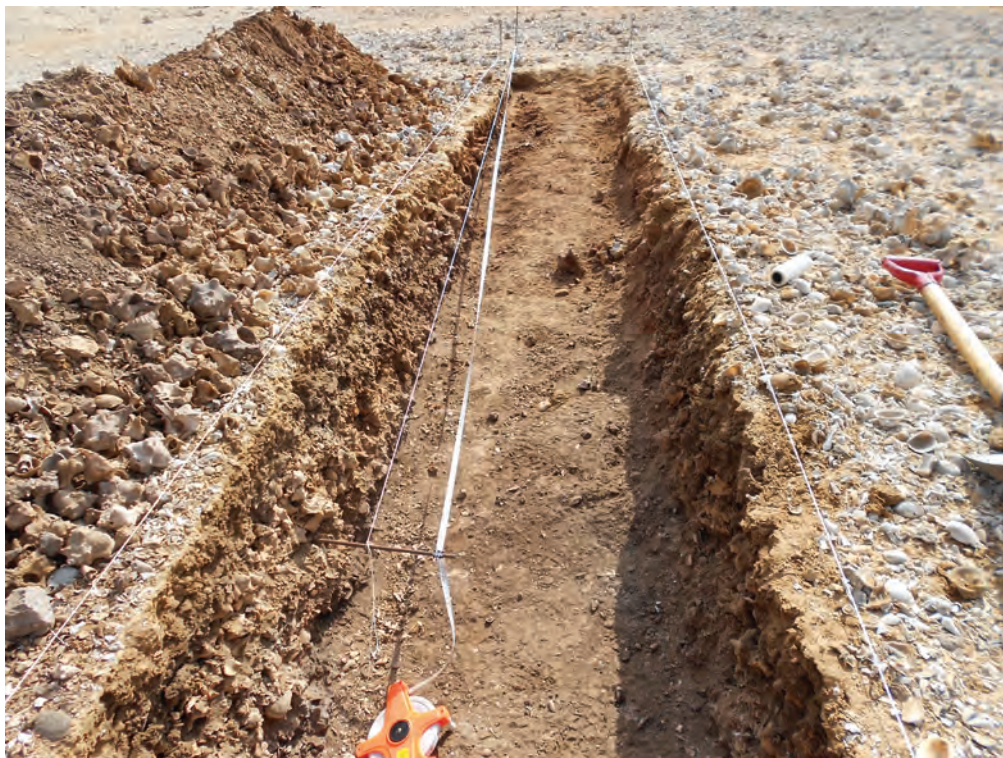
Figure 4.11. General view of JE5642 excavated trench, looking east. Photo by Niklas Hausmann, 25 January, 2013.
