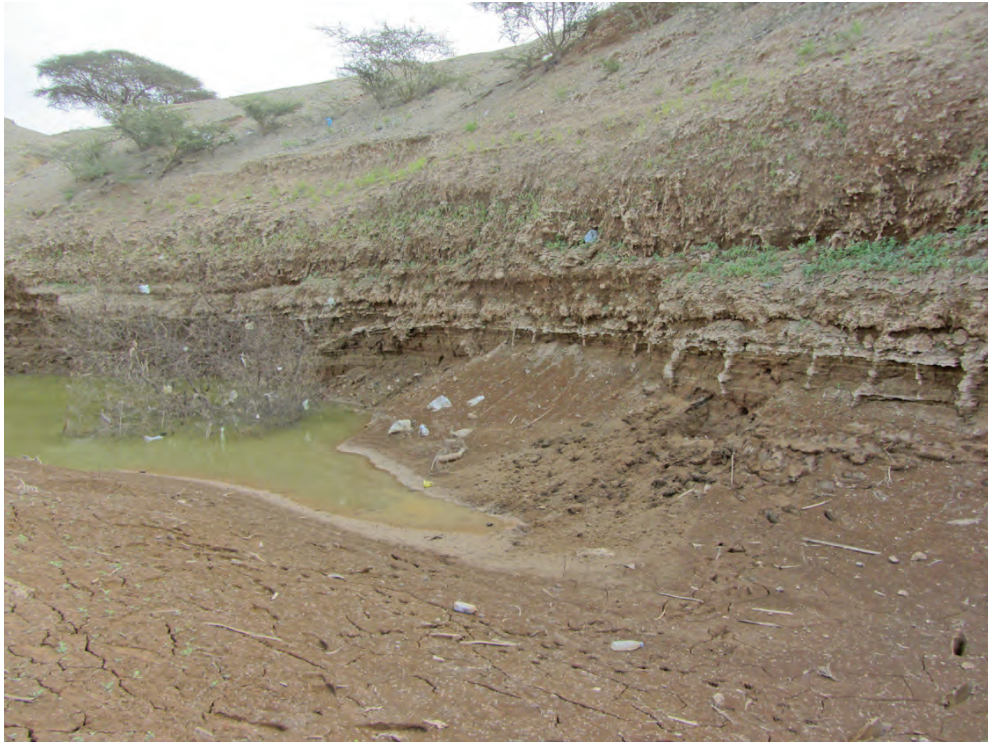
Figure 7.23: Hajambar Quarry in 2014 following flooding. The previously sampled section through the laminated wadi overbank sediments is behind the semi-submerged tree. The section cleaned and sampled for OSL dating is visible at the centre right of the photo. Photo: R. Inglis.
